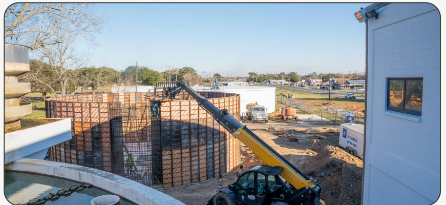
Water Plant Project: City secured $10.4 million in outside funding.
